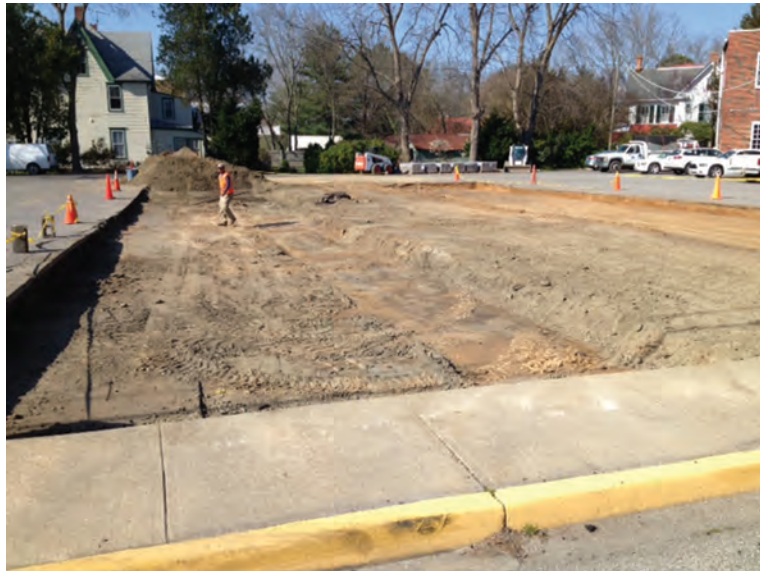
Figure 3.8. Excavation of permeable paver installation in small parking lot
