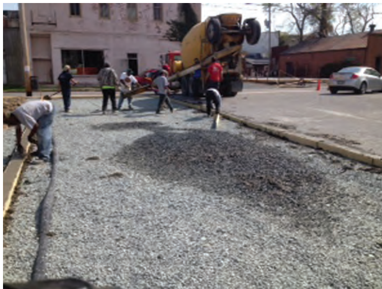
Figure 3.9. Installation of gravel reservoir layer
